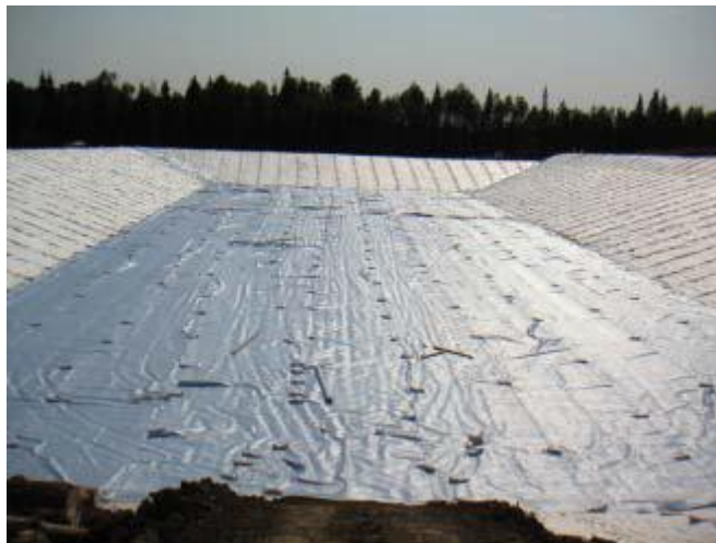
Figure 3: Secure landfill with synthetic liner
