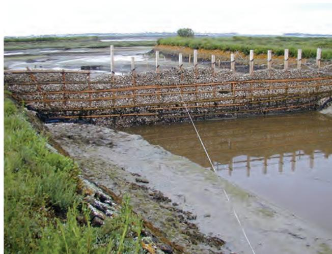
▲ *Figure 21: Barrier constructed from oyster-shells, held in place by stakes and nets.*
