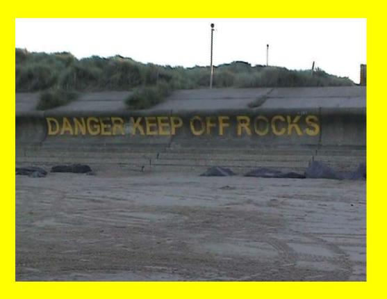
Advantages: It protects the foot of the cliff form erosion and can also prevent flooding.
